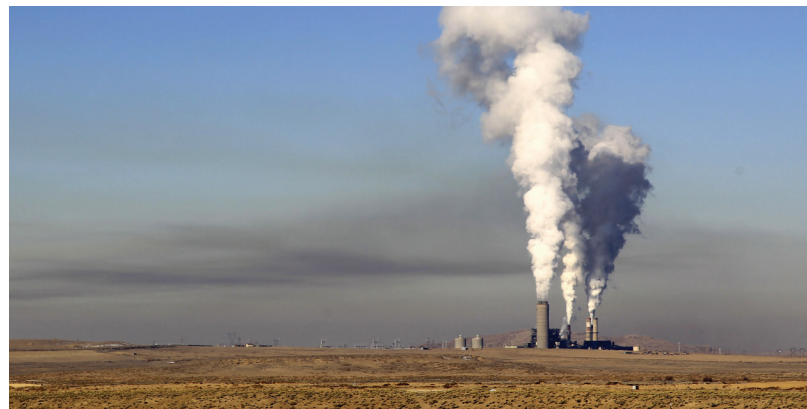
The Four Corners Generating Station operates on Navajo Nation land in New Mexico, producing coal-fired power for the region.
