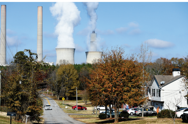
Plant Bowen, one of the largest coal-fired power plants in North America, rises behind a residential street in Bartow County, Georgia.
