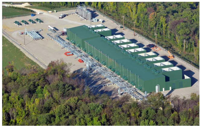
Compressor station complex: Compressors pressurize the gas to move it along in pipelines.
